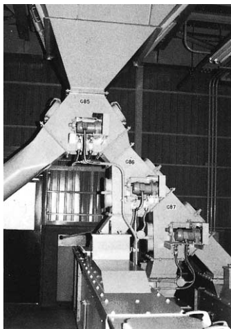
One-touch inspection doors installed on the two way gate
