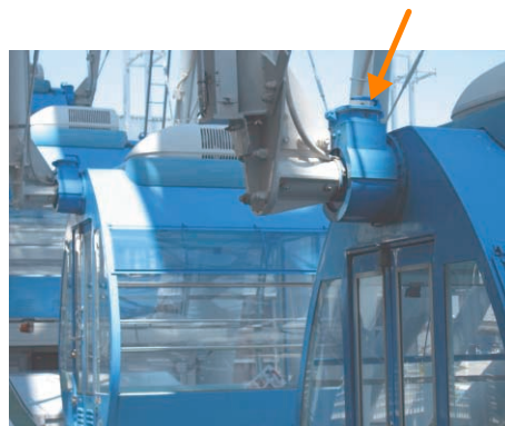
One-touch inspection doors installed on bearings of a Ferris wheel for inspection and lubrication
